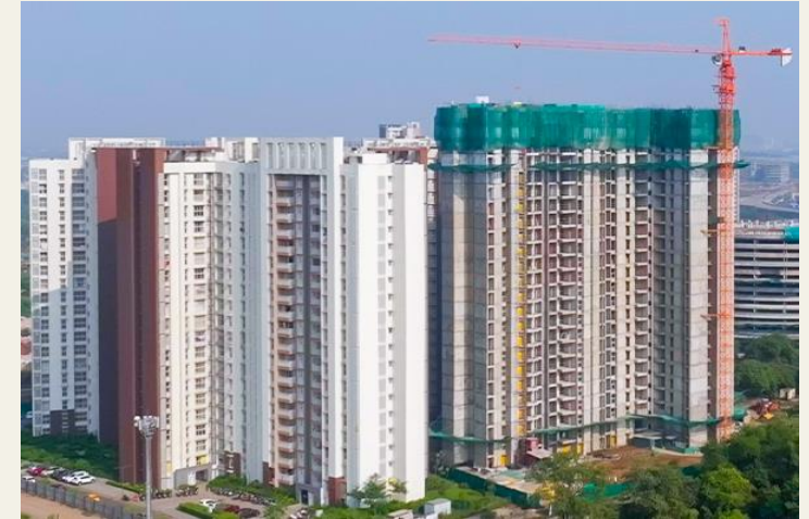
Use of low-carbon concrete mixes
