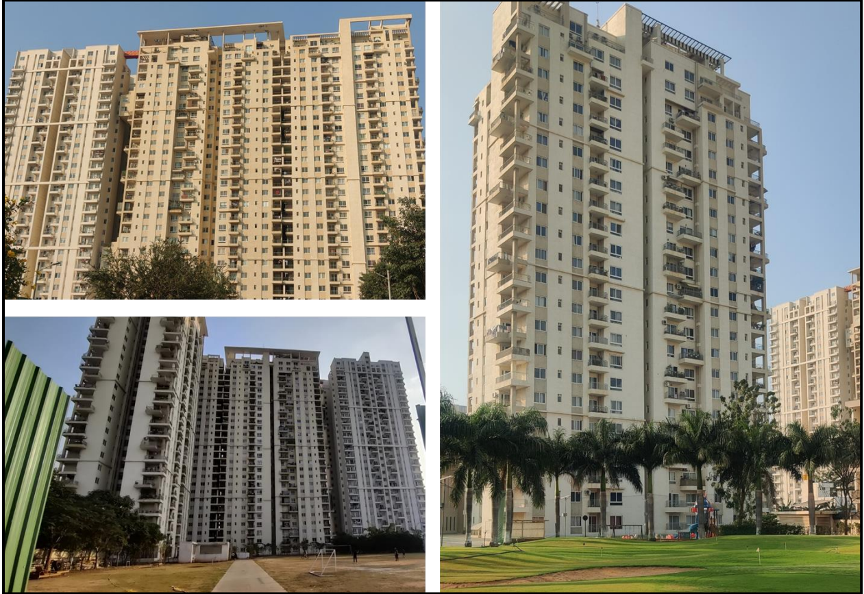
Photos: Completed Blocks of the Project
